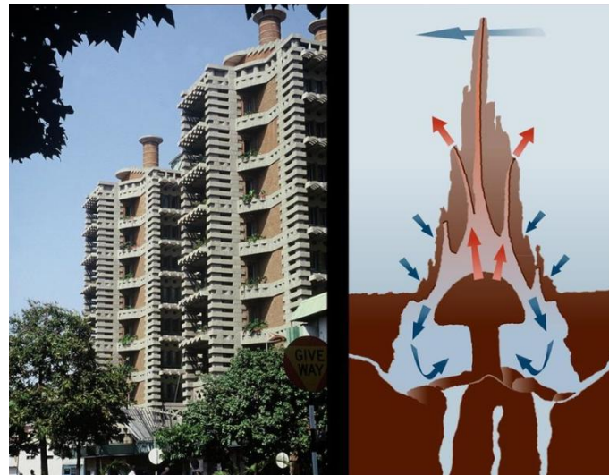
Fig. 20. Implementing the design principles of termite mounds to achieve natural ventilation in the Eastgate Center [5, 8].
